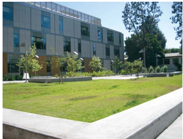
Retention Pond at Allied Health & Sciences Center
