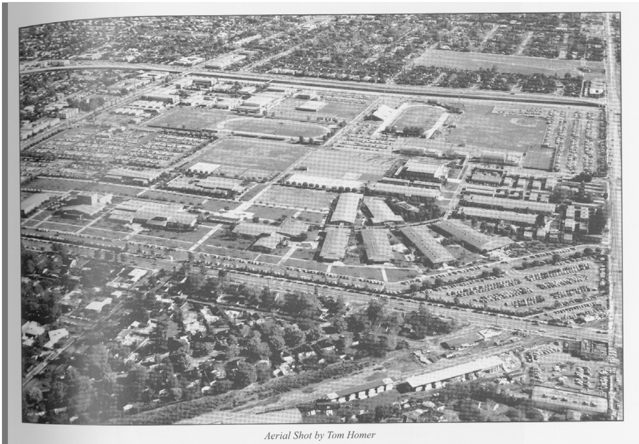
Figure A 1-1. Most buildings and plantings are in place by the late 1960s. Courtesy of "55 Years at Valley College: A Photo Retrospect"
