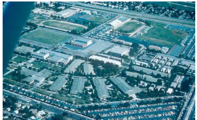
Figure A 2-5. This aerial view from around 1980 shows the maturing urban forest.
