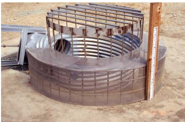
Figure 1 Example of Extended Detention Outlet Structure
